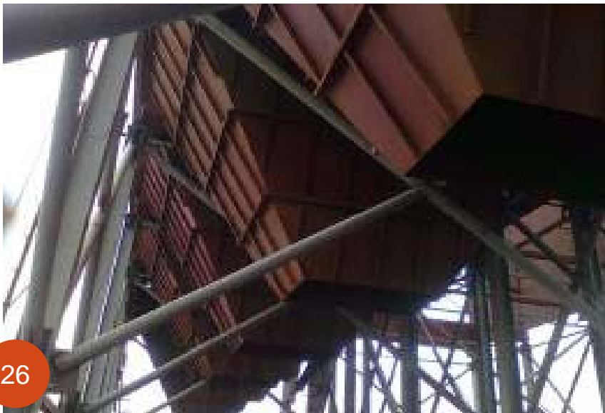
BTG Package: ESP#1: Hooper erection under progress
