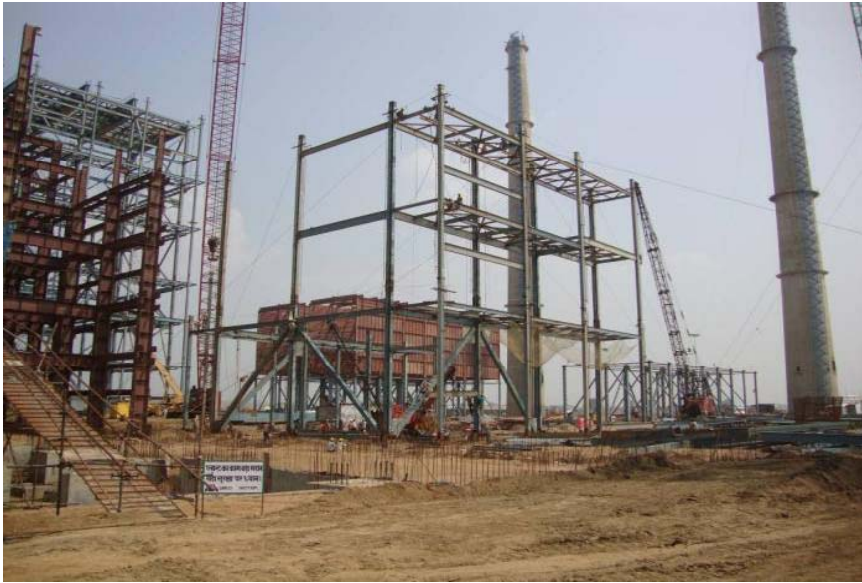
Erection of Boiler #2 columns
