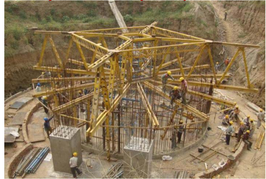
Reinforcement & Shuttering work for TG#2 Deck slab
